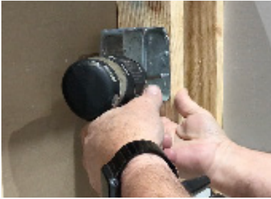
1. Mount a 4.0 or 3.5 (square or octagon) Junction Box flush to a wood or metal stud
