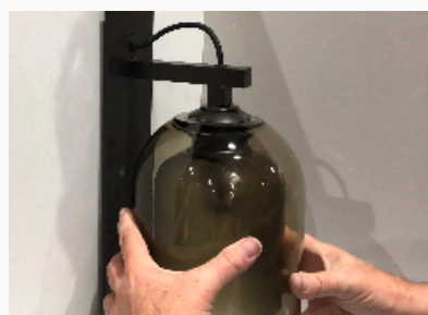
11. Attach the shade and install light globe
