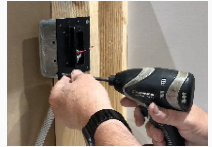
3. Attach the Mounting Plate to the Junction Box, center hole on top
